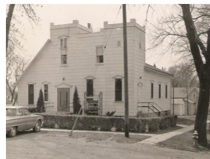
The same building was moved into the town of Arthur in 1943, and remodeled in 1949
